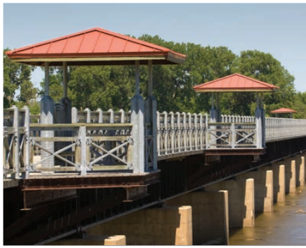
LIED PLATTE RIVER BRIDGE
